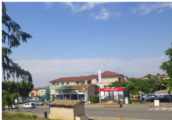
1 - La station service
